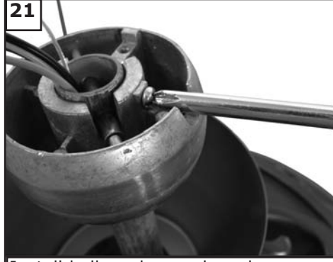
Install ball on downrod, replace cross pin and tighten screw securely.
