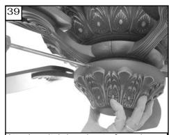
Attach switch housing to fan using the three screws provided.
