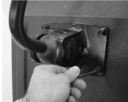
(2) Attach Omnimount plate to enclosure
