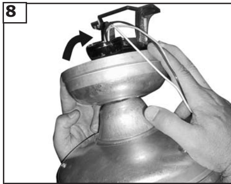
8 Carefully lift fan assembly onto mounting bracket. Rotate fan so that the notch on the ball engages the ridge in the mounting bracket. This will allow hands-free wiring.
