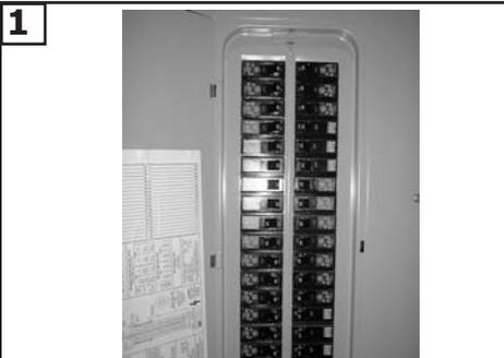
**1** Before you begin installing the fan, Switch power off at Service panel and lock service disconnecting means to prevent power from being switched on accidentally. When the service disconnecting means cannot be locked, securely fasten a prominent warning device, such as a tag, to the service panel.
