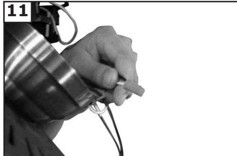
11 Make wire connections to power source using wire nuts provided. Make sure that no filaments are outside of the wirenut. After making the wire connections, the wires should be spread apart with the grounded conductor and the equipment-grounding conductor on one side of the outlet box and ungrounded conductor on the other side of the outlet box.
