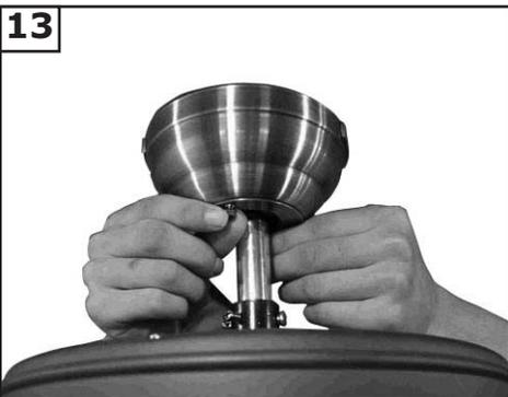
13 Next lift the canopy disk and install knurled nuts as shown. Tighten the knurled nuts securely. The canopy should adjust for any irregularity in the ceiling or Outlet box.
