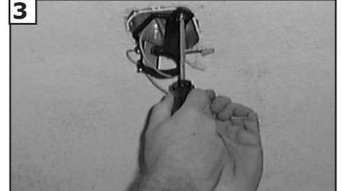
**3** Use metal outlet box suitable for fan support and use only the screws provided with the outlet box (must support 35 lbs). Before attaching fan to outlet box, ensure the outlet box is securely fastened by at least two points to a structural ceiling member ( a loose box will cause the fan to wobble). **Use only the screws provided with the outlet box.**
