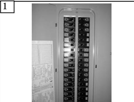
1 Before you begin installing the fan, Switch power off at Service panel and lock service disconnecting means to prevent power from being switched on accidentally. When the service disconnecting means cannot be locked, securely fasten a prominent warning device, such as a tag, to the service panel.
