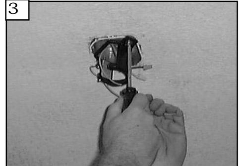
3 Install the Mounting Bracket to the Outlet box. Use only the screws provided with the outlet box.
