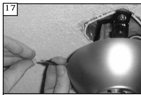
17 Make wire connections to power source using wire nuts provided. Make sure that no filaments are outside of the wirenut. After making the wire connections, the wires should be spread apart with the grounded conductor and the equipment-grounding conductor on one side of the outlet box and ungrounded conductor on the other side of the outlet box.
