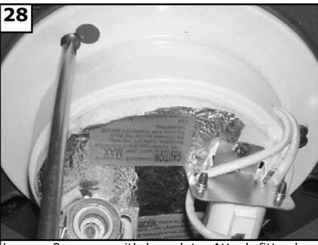
Loosen 3 screws with key slots. Attach fitter by placing over screws and twisting clockwise into place. Tighten all 3 screws securely.
