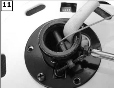
11 Loosen 2 screws and remove pin with keeper for downrod, yoke cover and canopy to fit in yoke of fan.
