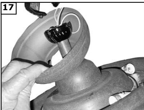
17 Raise fan with downrod assembled to the ceiling bracket and hang fan assembly. Be sure to rotate the downrod ball so that the notch in the bracket engages the slot in the ball.
