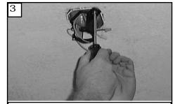
Use metal outlet box suitable for fan support (must support 35 lbs). Before attaching fan to outlet box, ensure the outlet box is securely fastened by at least two points to a structural ceiling member ( a loose box will cause the fan to wobble). Use only the screws provided with the outlet box.
