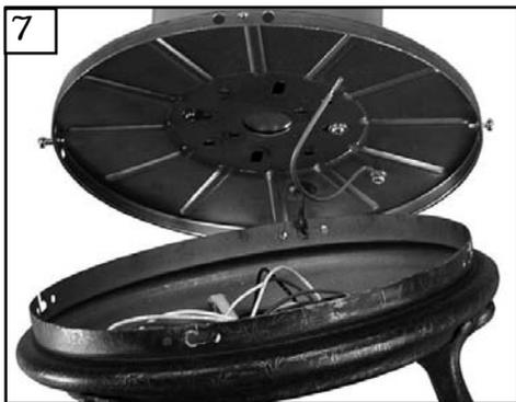
7 Hang fan from hook on the mounting plate. Use the closed hole. This will allow for hands free wiring.
