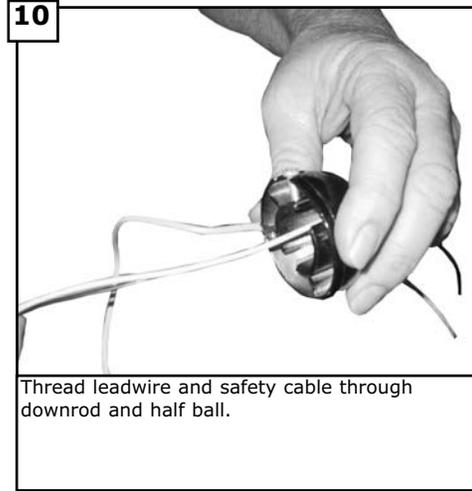
Thread leadwire and safety cable through downrod and half ball.
