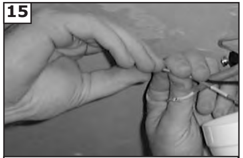
15 Make wire connections to power source using wire nuts provided. Make sure that no filaments are outside of the wirenut. After making the wire connections, the wires should be spread apart with the grounded conductor and the equipment-grounding conductor on one side of the outlet box and ungrounded conductor on the other side of the outlet box.
