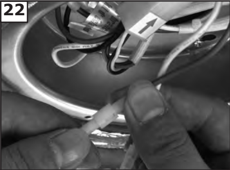
22 Connect white wire from fan to white wire from light fixture. Then plug blue wire from fan to black wire from light fixture.
