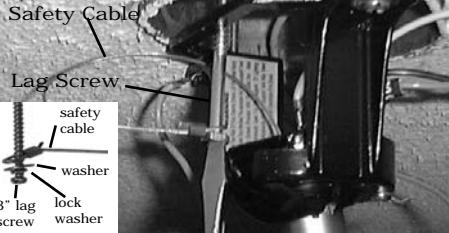
Fan and light kit combinations over 35 lbs, in both flush and downrod mode the safety cable must be installed into the house structure beams using the 3" lag screws, washers, and lock washers, provided. Make sure that when the safety cable is fully extended the lead wires are longer than the cable and no stress is placed on the lead wires.
