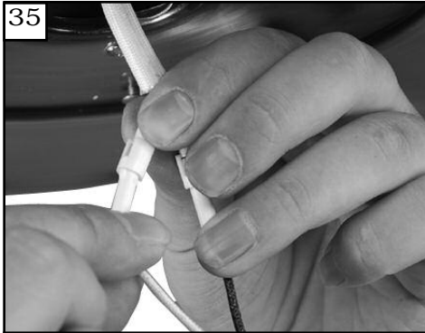
35 Plug white wire from fan to white wire from light kit. Then plug black wire from fan to black wire from light kit.
