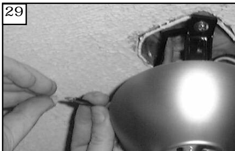
29 Make wire connections to power source using wire nuts provided. Make sure that no filaments are outside of the wirenut. After making the wire connections, the wires should be spread apart with the grounded conductor and the equipment-grounding conductor on one side of the outlet box and ungrounded conductor on the other side of the outlet box.
