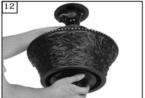
Raise fan with downrod assembled to the ceiling bracket and hang fan assembly. Be sure to rotate the downrod ball so that the notch in the bracket engages the slot in the ball.
