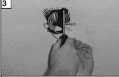
Use metal outlet box suitable for fan support (must support 35 lbs). Before attaching fan to outlet box, ensure the outlet box is securely fastened by at least two points to a structural ceiling member ( a loose box will cause the fan to wobble). **Use only the screws provided** with the outlet box.
