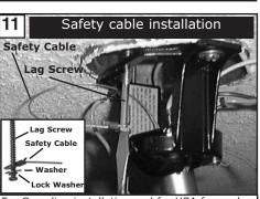
For Canadian installation and for USA fan and light kit combinations over 35 lbs, in both flush and downrod mode the safety cable must be installed into the house structure beams using the 3" lag screws provided. Make sure that when the safety cable is fully extended the leadwires are longer than the cable and no stress is placed on the leadwires.
