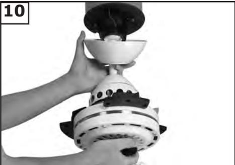
**10** Hang assembled fan from the mounting bracket installed to ceiling in previous step. Make sure the fan is hanging straight. Rotate fan until the tab on the Mounting bracket engages the slot on the Downrod Ball. This must be done to prevent the fan body from rotating when the blades are in motion.
