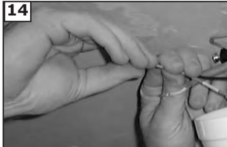
**14** Make wire connections to power source using wire nuts provided. Make sure that no filaments are outside of the wirenut. After making the wire connections, the wires should be spread apart with the grounded conductor and the equipment-grounding conductor on one side of the outlet box and ungrounded conductor on the other side of the outlet box.
