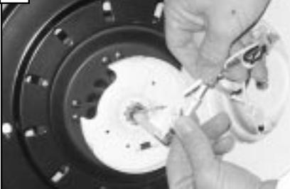
Plug in electrical connection from fan into the connectors on fitter.
