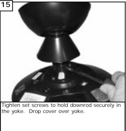
Tighten set screws to hold downrod securely in the yoke. Drop cover over yoke.
