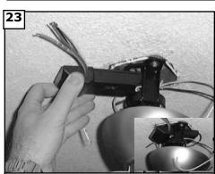
Install remote receiver by sliding into opening in the Mounting bracket. Make sure that the dip switches on the Transmitter and the Receiver are set to the same position. See Fig 31 for remote operation
