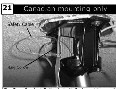
For Canadian installation in both flush and downrod mode the safety cable must be installed into the house structure beams using the 3" lag screws provided. Make sure that when the safety cable is fully extended the leadwires are longer than the cable and no stress is placed on the leadwires.
