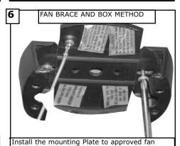
brace and box combination use only the hardware provided with the fan brace and box.
