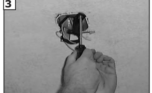
**3** Use metal outlet box suitable for fan support (must support 35 lbs). Before attaching fan to outlet box, ensure the outlet box is securely fastened by at least two points to a structural ceiling member ( a loose box will cause the fan to wobble). **Use only the screws provided with the outlet box.**
