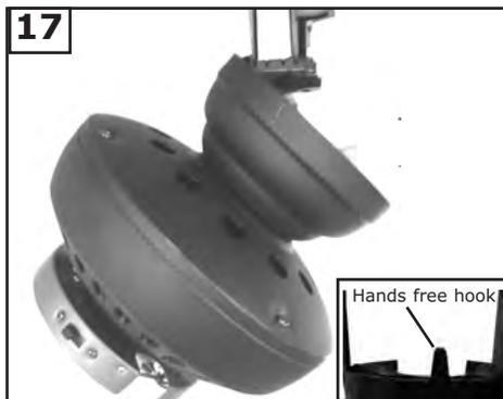
17 Hang fan from mounting bracket by the hands free hook into a closed hole on the edge of the Canopy. Note: For Canadian mounting refer to Step #8.
