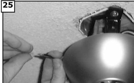
25 Make wire connections to power source using wire nuts provided. Make sure that no filiments are outside of the wirenut. After making the wire connections, the wires should be spread apart with the grounded conductor and the equipment-grounding conductor on one side of the outlet box and ungrounded conductor on the other side of the outlet box.
