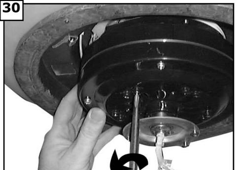
30 Remove motor screws from fan motor and save.
