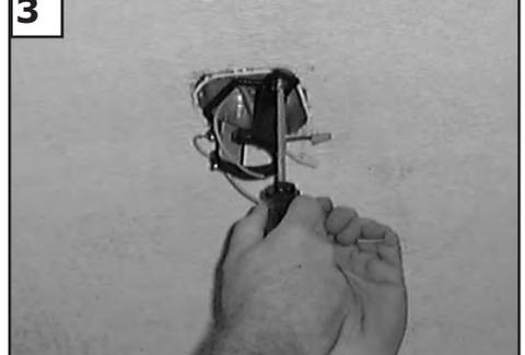
Install the Mounting Bracket to the Outlet box. **Use only the screws provided with the outlet box.**
