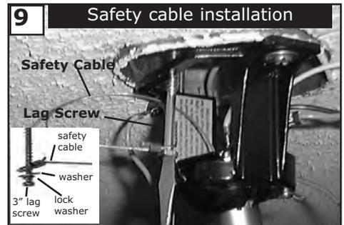
For Canadian installation and for USA fan and light kit combinations over 35 lbs, in both flush and downrod mode the safety cable must be installed into the house structure beams using the 3" lag screws, washers, and lock washers provided. Make sure that when the safety cable is fully extended the leadwires are longer than the cable and no stress is placed on the leadwires.
