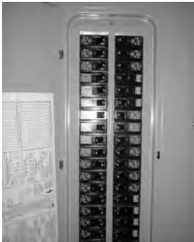
Before you begin installing the fan, Switch power off at Service panel and lock service disconnecting means to prevent power from being switched on accidentally. When the service disconnecting means cannot be locked, securely fasten a prominent warning device, such as a tag, to the service panel.
