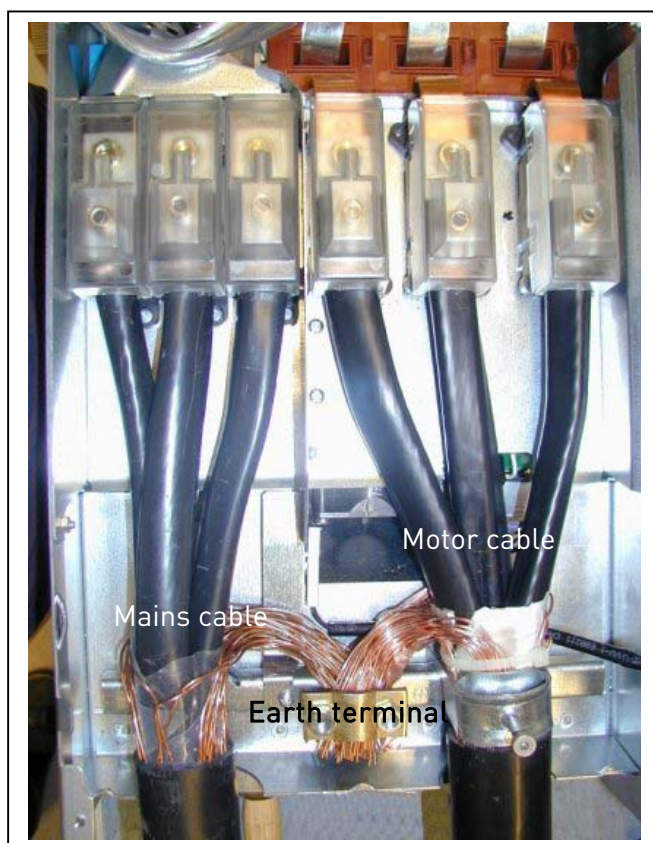
Figure 6-16. Cable installation in Vacon NX, FR8
