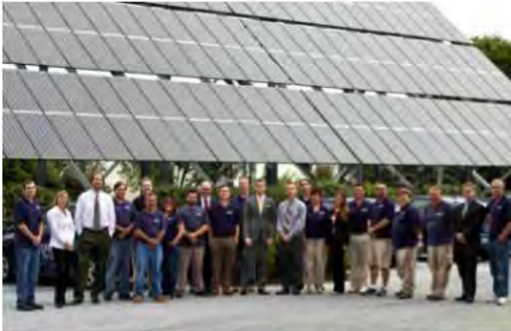
Haverford Systems is 100% Solar Powered.
