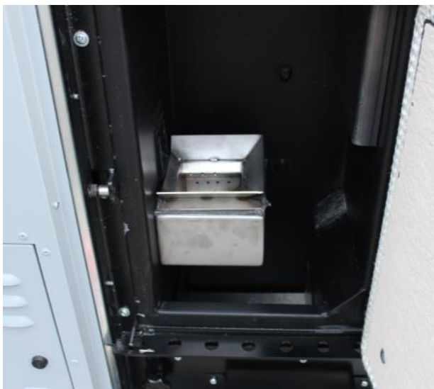
Always allow boiler to cool down before opening the combustion chamber door.
