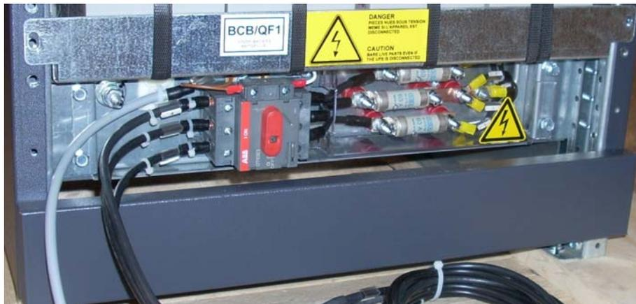
Picture 25 – Battery circuit breaker and fuses
