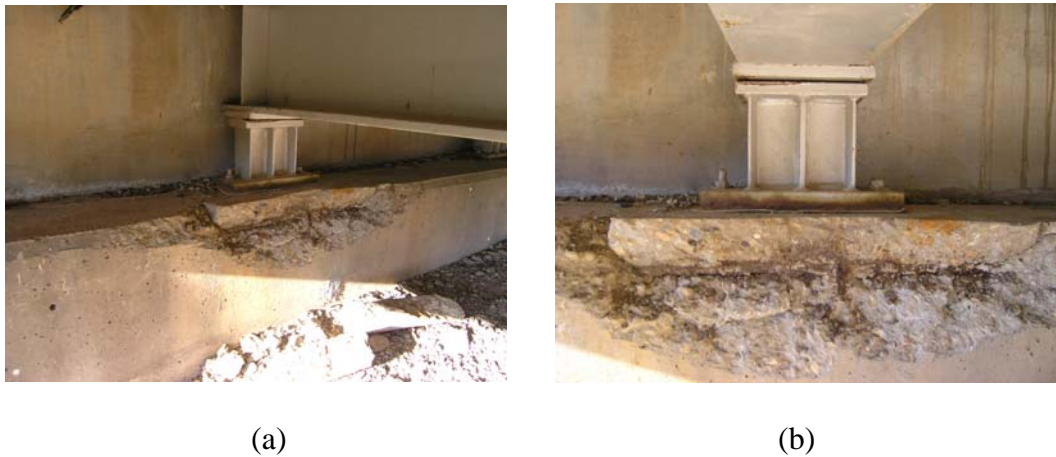
FIGURE A8 Spall with Exposed Rebar at Abutment: (a) Poor and (b) High Quality Picture.
