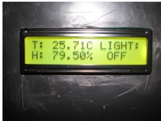
Figure 4.8 : Light condition is OFF
