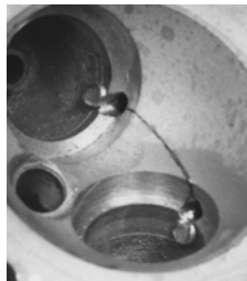
Drill Holes for Plugs
