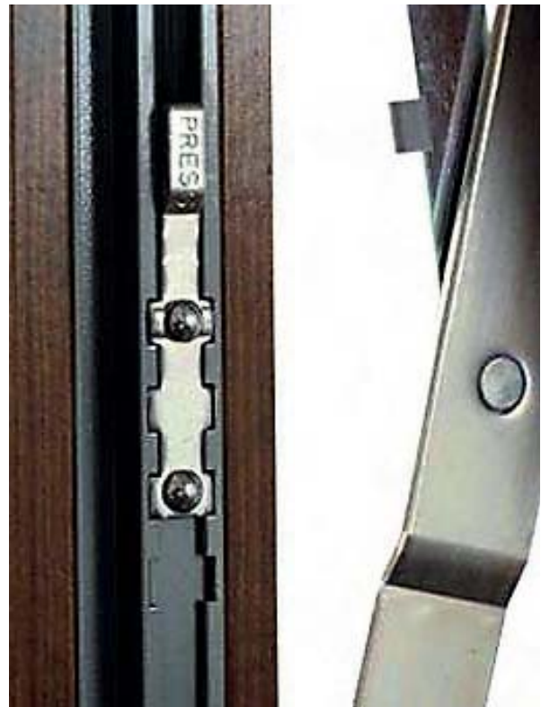
Figure 1.7. Catcher for an LW11 top swing window
