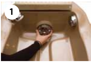
1 Remove suction cover by turning counter-clockwise.
