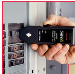
The Circuit Breaker Identifier Model CBI-1 receiver scans a power panel.
