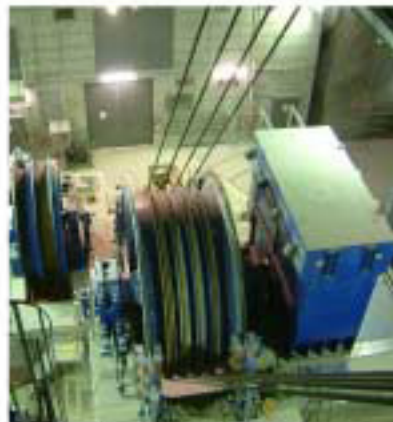
New mine hoist systems – p4
