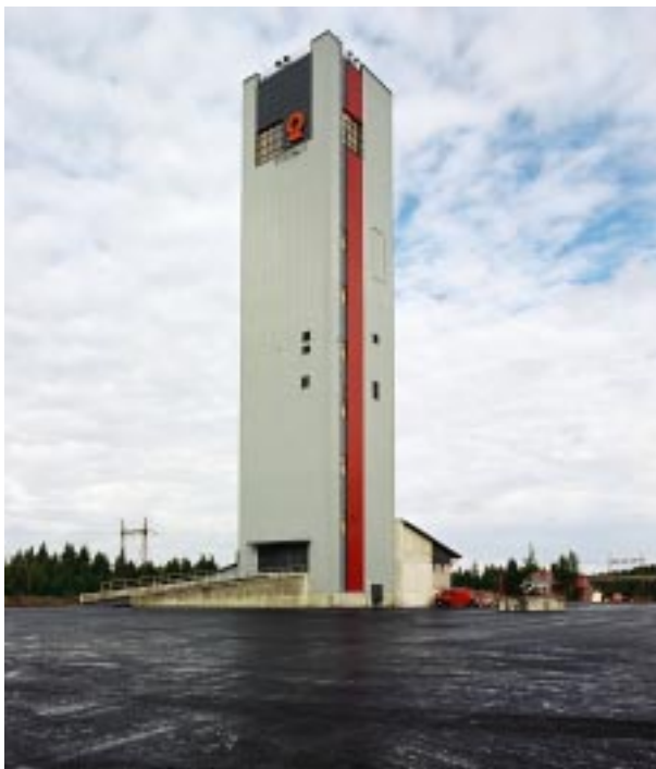
The headframe of the Pyhasalmi Mine in Finland.
