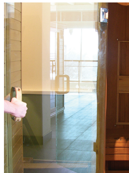
You may have to partially close the door to line up with the bottom hinge
