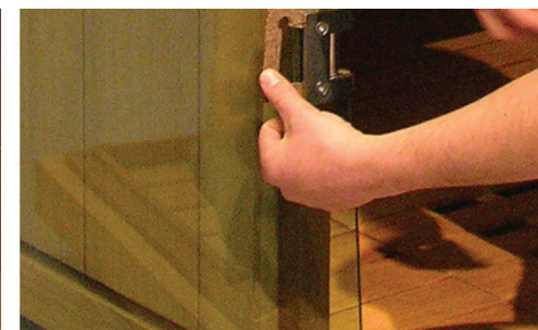
Slide gaskets in place
