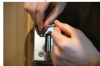
Hex tool tightens hinge
