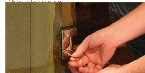
Tighten hinge with hex tool
