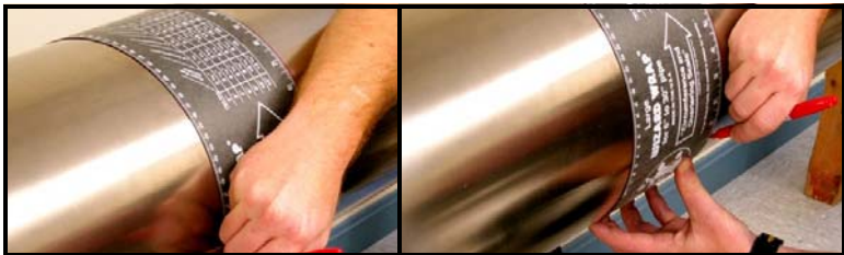
Figure 3-5: Measuring and Marking Circumference Lines
