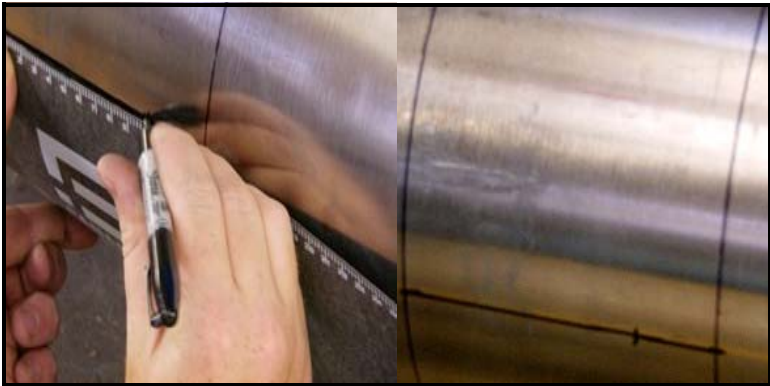
Figure 3-15: Marking the 9 o'clock Position
