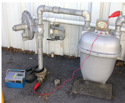
(Correct - Bridging cable attached around the insulator bridges the break in the conductor loop)
