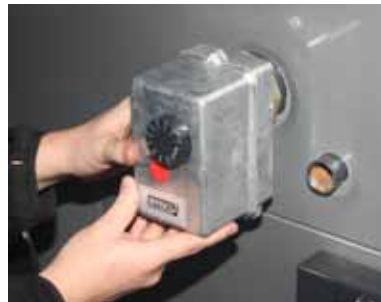
2. Installation of the thermostat
