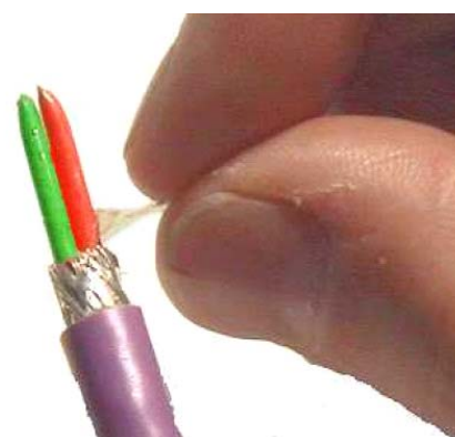
Cable terminal processing
