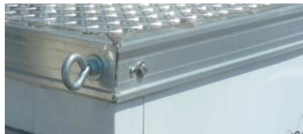
Eye bolt tie-downs to stabilize platform in windy conditions
