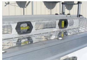
Carpenter's Level on rooftop to level
