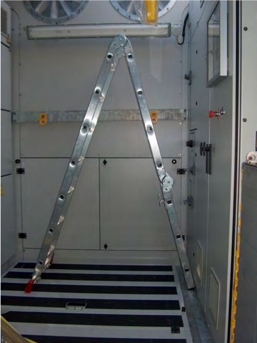
Picture 8 Ladder to roof
