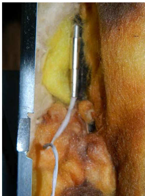
Fig. 2 Insulate around RTD and
