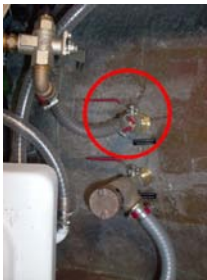
Seawater intake valve (Reference 2)
