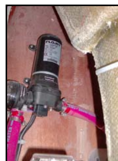
Pump for deck washing - 12V (Reference 3)
