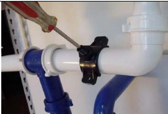
Align the drilled hole in the drain pipe with the drain saddle using a drill bit or narrow screwdriver
