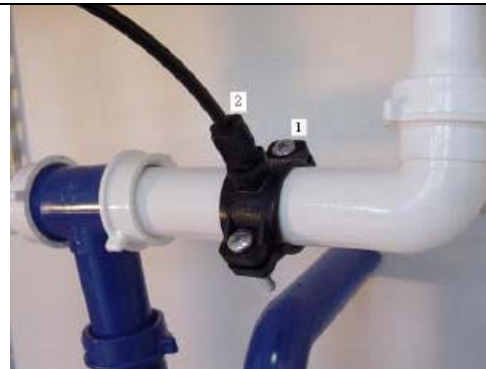
Put the complementary piece and clamp them together with the two bolts. (1) Tighten the two bolts evenly (2) Connect tubing
