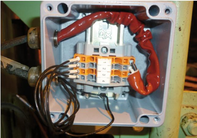
11. Push back the wiring in the silicone flex tube to a good position inside the junction box.
