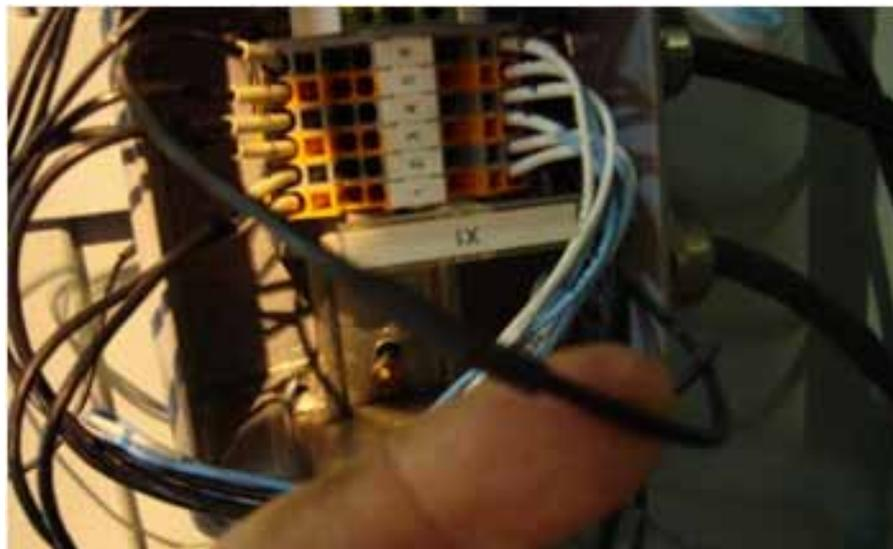
**Figure 13:** The wire after shrink tube has been used to cover the insulation failure. Additional repair will include making sure the wires are well supported and don't touch the junction box.
