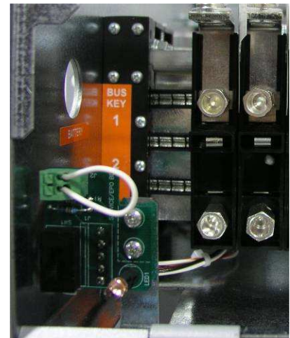
Figure 18 - EPO and Service Bypass Switch in 23" 6U Distribution
