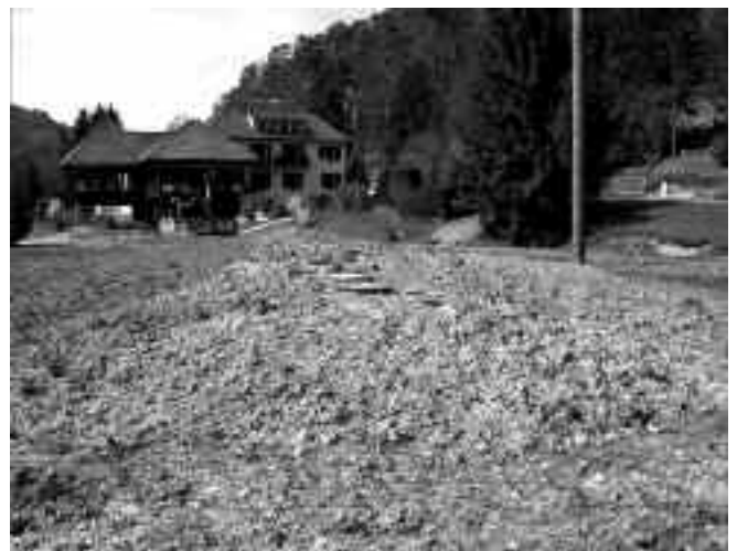
Arnsbourg at Baerenthal (F-57). Semi-buried placement, finished with topsoil and reseeded with grass
