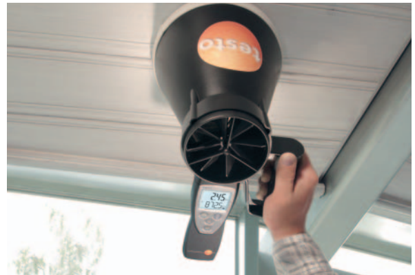
testo 417 monitoring the air flow at a ventilation duct
