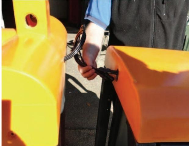
Figure 8. Inserting air lines.
