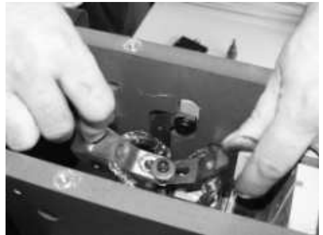
Fig. 52-4 Replace arcing contact
