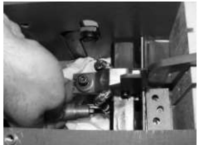
Fig. 52-4 Replace arcing contact
