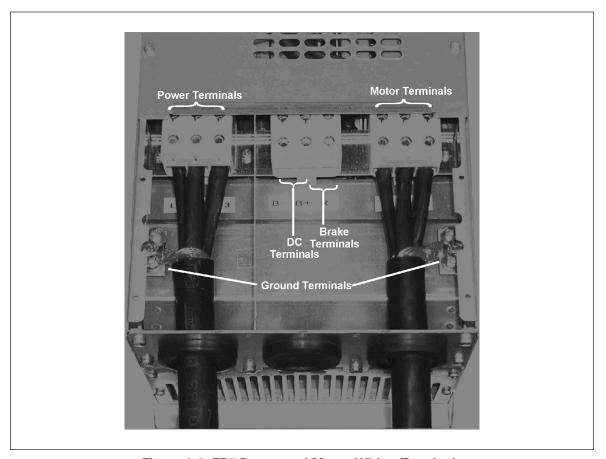
Figure 3-2: FR7 Power and Motor Wiring Terminals
