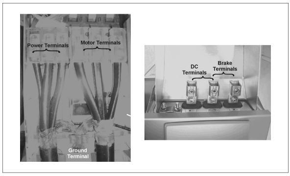
Figure 3-3: FR8 Power and Motor Wiring Terminals
