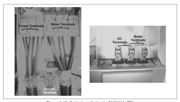
Figure 3-15: Cable Installation in SLX9000, FR8
