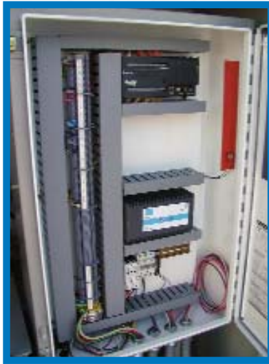
Enclosure containing DL06 PLC, Rhino power supply, and Cutler-Hammer motor controls.
